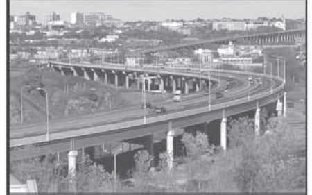
NJ Turnpike East Viaduct
