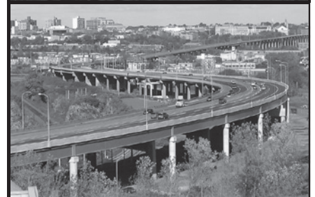
NJ Turnpike East Viaduct
